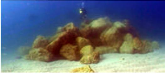
*Figure 13: Piles of natural limestone boulders can be used to create an artificial reef. Natural boulders can be drilled to accept coral adapter plugs for coral rehabilitation projects. From our experience we recommend that boulders be at least 3 tons, and be deployed in a stable configuration, in order to prevent shifting in storms.*
