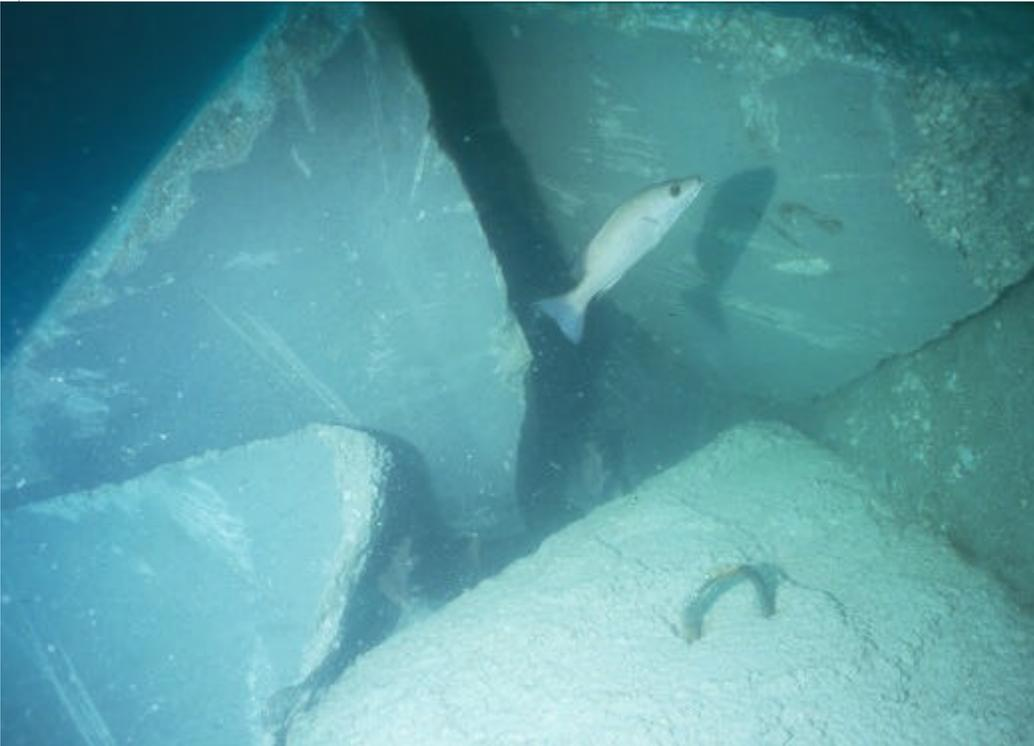
*Figure 12: Solid concrete tetrahedral blocks used as an artificial reef. Solid blocks do not create as much void space as hollow designs, but if deployed properly, can be extremely stable.*
