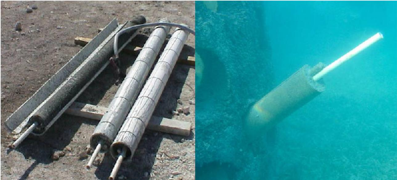
Figure 23: Battered pile anchors before (left) and after (right) installation. Battered piles are used in groups of three or four, to resist both horizontal and vertical movement in areas with soft sediment.
