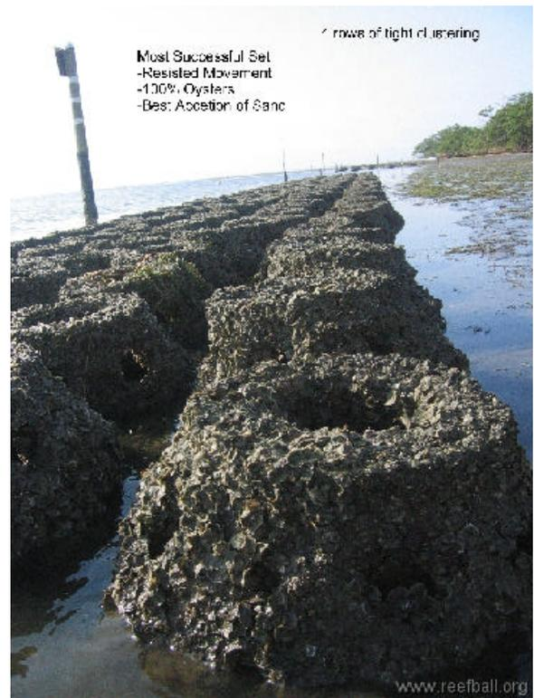
Figure 0 Shoreline stabilization project with oyster recruitment, MacDill Air Force Base, Florida. Photo: Reef Ball Foundation.
