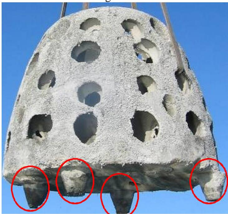
*Figure 21: Anchoring cones (circled in red) can be used to prevent horizontal movement in soft to semi-firm bottoms. Cones are cast monolithically when the Reef Ball is made, and designed to settle slowly into the ocean bottom. Once settled, the cones will prevent lateral movement during storms*
