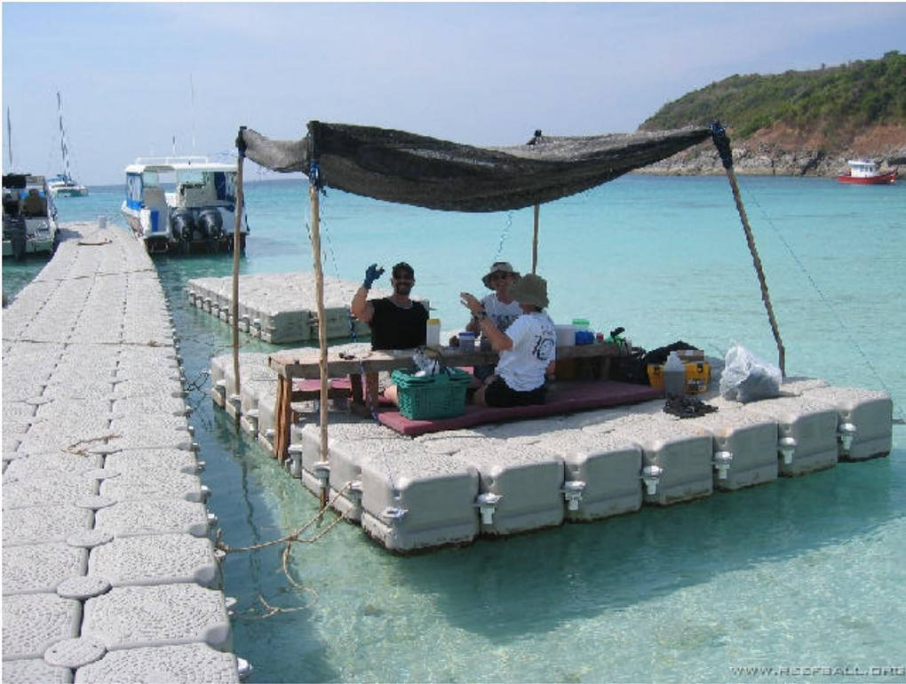
Figure G17: Floating coral table. Floating tables are ideal for use in most low energy locations, are more comfortable for the table workers, and automatically adjust for factors such as tides. If resources and conditions permit, consider the construction of a floating table.
