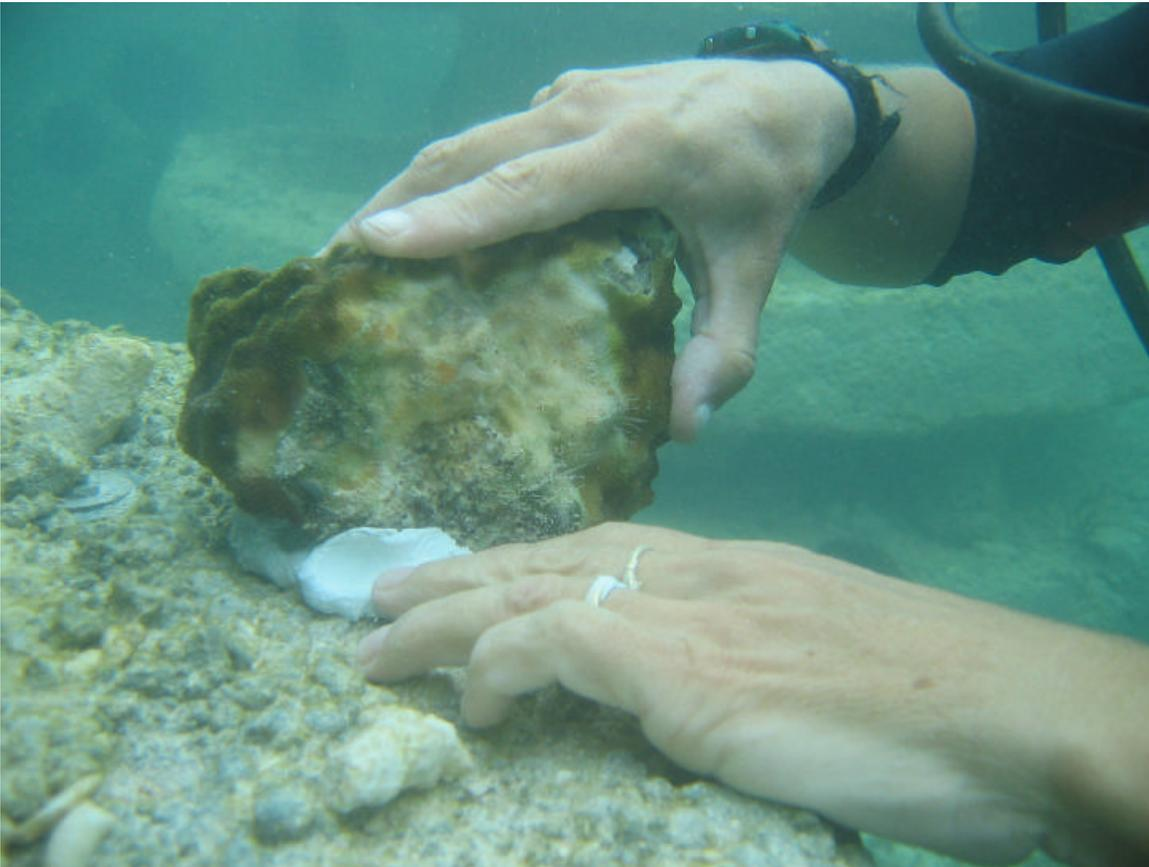
*Figure G19: Diver using the direct putty method to attach a rock to a base substrate unit using epoxy putty. This method is used primarily for aquascaping- the process of putting the finishing aesthetic touches on a project*
