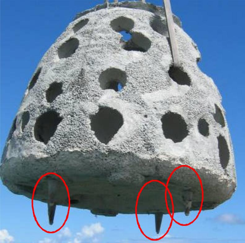
*Figure 21: In areas with hard packed bottom, pre-cast concrete spiked with #5 fiberglass rebar reinforcement can be used in place of anchoring cones. They serve the same purpose as anchoring cones, but can penetrate firmer bottom.*
