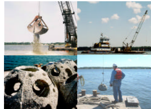
Mill Hill Oyster Sanctuary Installation & Field Test
