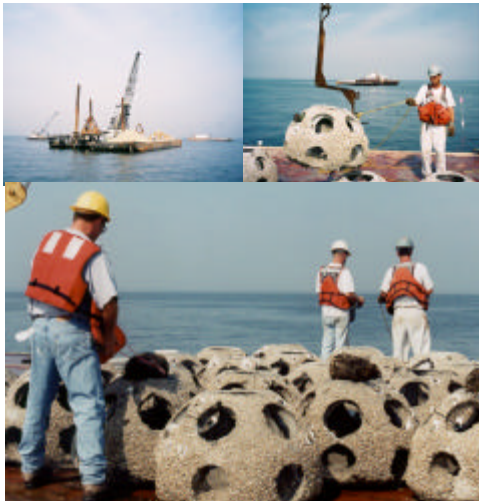
Memorial Reef Installation & Technology Field Test
