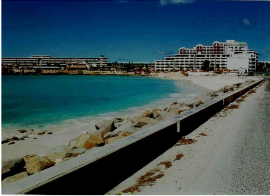
Figure 3. Wall and rocks along road at end of runway (photo date unknown).
