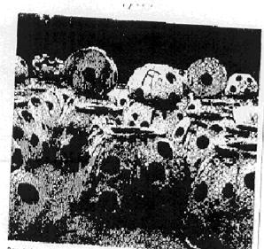
Ready for deployment to a coastal fishing site, concrete spheres known as reef balls attract fish by providing hires of hideouts on an otherwise featureless sea floor.
