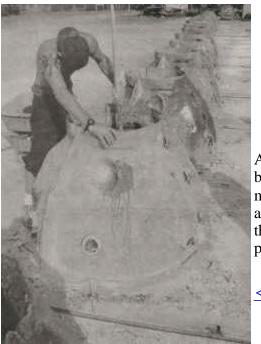
A WORKER for Reef Innovations, an artificial reef company based in Florida, prepared these pallet reef ball molds Monday morning by dumping dirt and sand inside the structures. The dirt and sand was said to prevent the concrete from leaking out of the bottom of the molds when it is poured over them. (N. Garrett photo)
