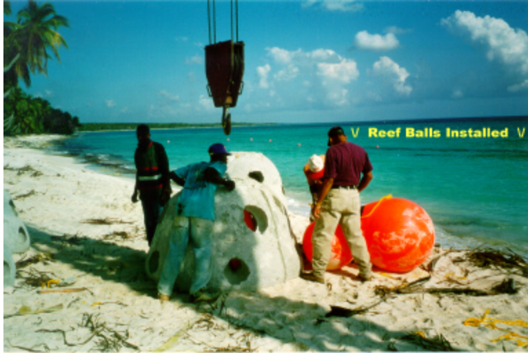
Ultra Reef Balls being deployed at Gran Dominicas Hotel in the Dominican Republic, note the appearance of the Reef Ball submerged breakwater as only a dark line in the water. This would be the same look generated at the Bahia Principe Tulum and Akumal Hotels.
