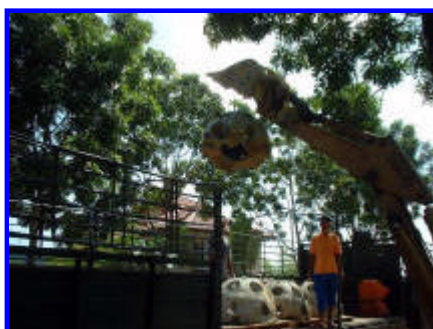
Hoisting high over the railings
