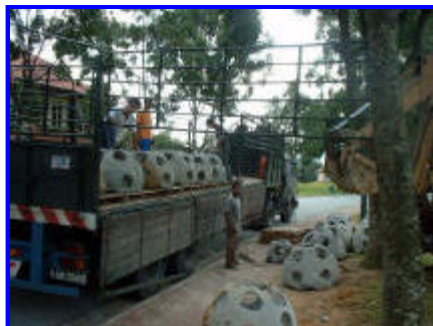
Reefballs are hoisted on to the trailer
