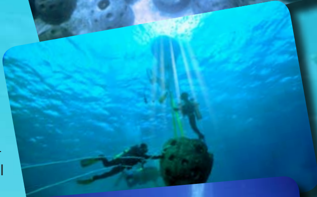
Liftbag was used to pull up the reefball
