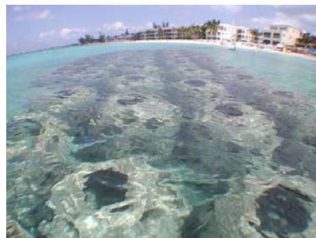
Figure 3 – Reef Ball Submerged Breakwater
