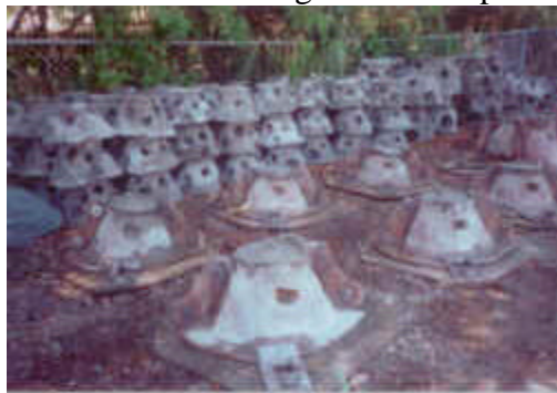
Molds used to construct the 100 reef units for installation in the Westshore area of Tampa.
