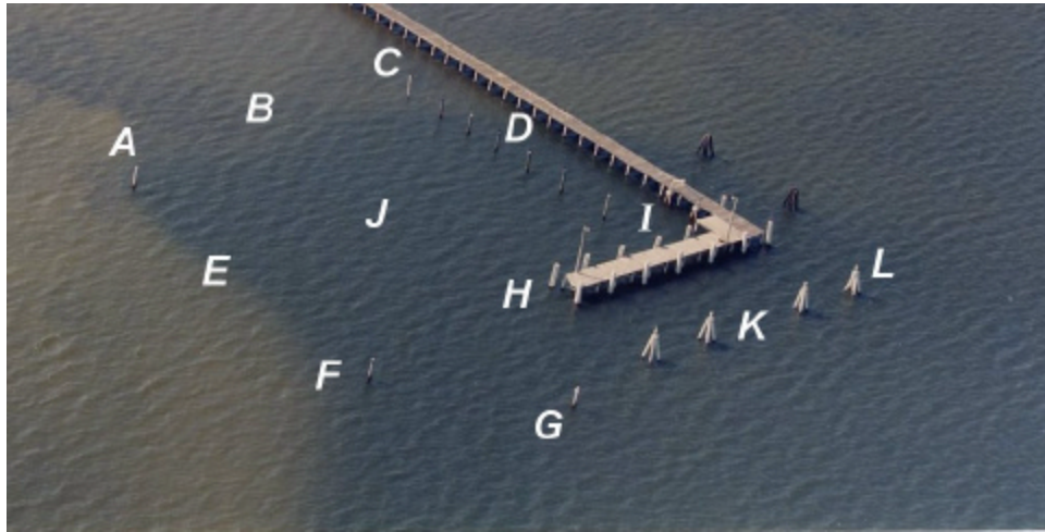
Figure 5. Designation of Points for Survey of Pier at Indian Riverside Park
