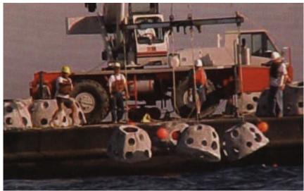
Resembling some strange offspring from outer space, the Reef Balls are towed to the site by barge, then lowered by sea-going crane to their final resting place.
