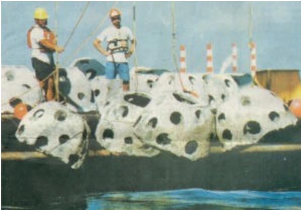
*GOING DOWN: Workers on a barge guide concrete 'reef balls' toward their- new home on a damaged reef about a quarter-mile off Dania Beach on Friday. Below, a crane on the barge helps lower the 160 balls.*
