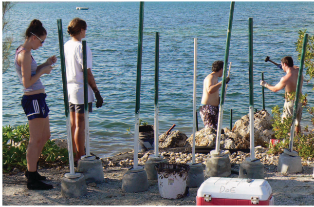
Figure 2. Project volunteers (left to right: Hannah Williams, Dr. Catherine Jadot, David Hudson, and Jason Krumholz) assist in deploying and collecting initial monitoring data for a pilot test of the “armored cultivator” high-energy mangrove restoration technique at the Cayman Islands Sailing Club in Grand Cayman, BWI. Cultivator units (foreground) are filled with local sediment, sealed with a slow-release fertilizer disc (shown on top of cultivators), and anchored in place so the top of the wrack tube is a few inches above the spring high-water level. Photo courtesy of www.reefball.com
