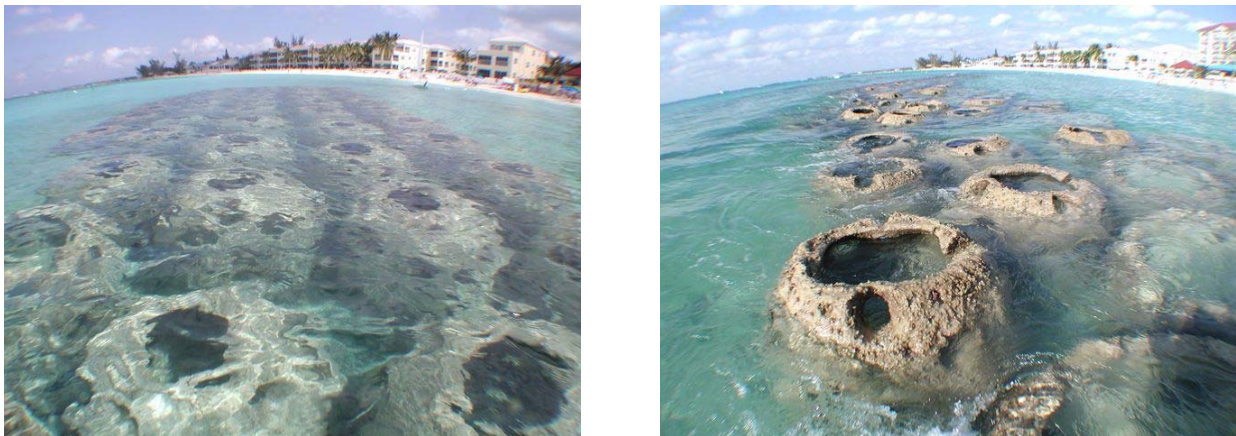
Figure 11. Northern (left) and Southern (right) Reef Ball Artificial Reef Submerged Breakwater Segments at Extreme Low Tide.
