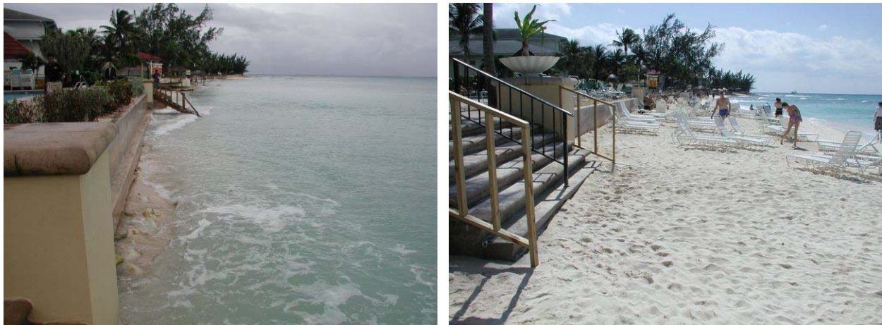
Figure 1. Before and After Breakwater Installation Photographs – View South October 2002 (left) and February 2003 (right)
