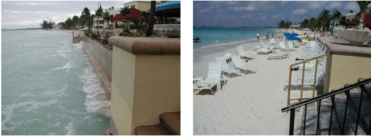
Figure 2. Before and After Breakwater Installation Photographs – View North
