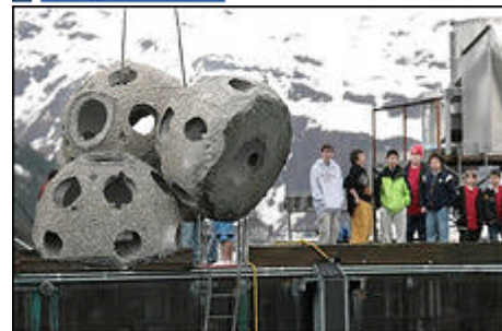
A group of school children watch as concrete balls weighing hundreds of pounds each, are lowered into the water at Smitty's Cove in Whittier, Alaska Wednesday May 10, 2006 to make Alaska's first artificial reef. The reef was in response to damage done when Alaska Marine Lines expanded its container facility at Whittier last year. (AP Photo/AI Grillo) (AI Grillo - AP)
